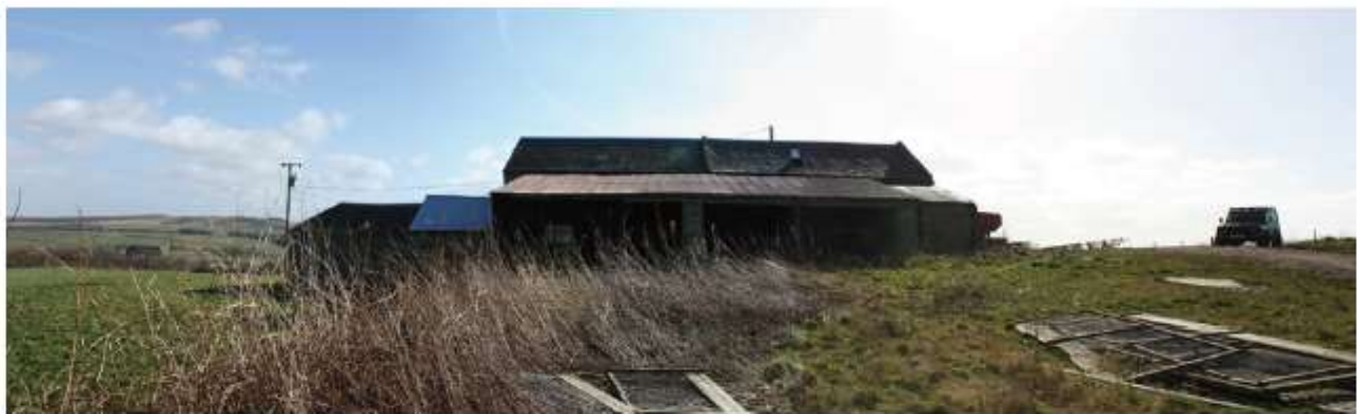
2. View of the Existing Stone Wall Agricultural Building on The Eastern Edge of the Site
